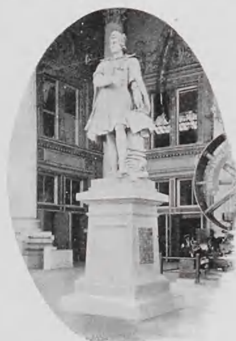
ENTRANCE TO MACHINERY HALL
